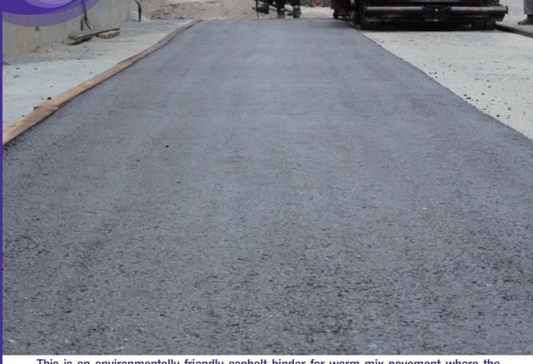
This is an environmentally friendly asphalt binder for warm mix pavement where the manufacturing temperature of the mixture has been suppressed.
